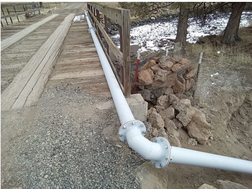
Steel pipe across canal bridge
