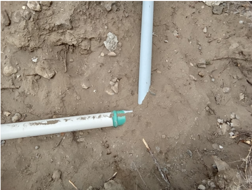
Connection to existing mainline from pump
