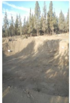
After: New pond and liner was constructed to eliminate flood irrigation.
