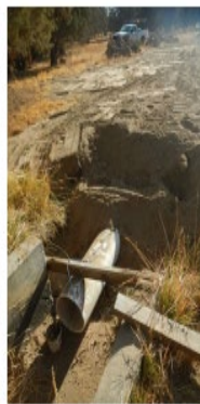
During Construction: Existing ditch was cleaned and set on grade. 10 inch PVC gasketed pipe was installed with 36 inch of soil cover over the pipe. Area was seeded to native seed.
