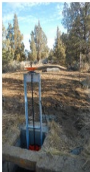
After: New headgate and concrete weir box structure (background).
