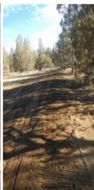
During Construction: Existing ditch was cleaned and set on grade. 10 inch PVC gasketed pipe was installed with 36 inch of soil cover over the pipe. Area was seeded to native seed.
