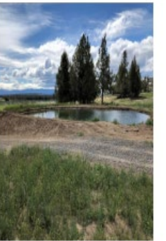
After: Completed Irrigation pond.
