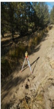
During Construction: Existing ditch was cleaned and set on grade. 10 inch PVC gasketed pipe was installed with 36 inch of soil cover over the pipe. Area was seeded to native seed.
