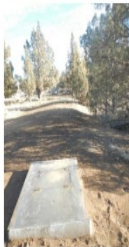
After: Close up of concrete weir box structure with safety lid.
